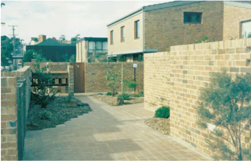
The residential development makes use of brick walls to create private living areas. The higher screen wall on the right provides shielding from traffic noise for an outdoor living area.
