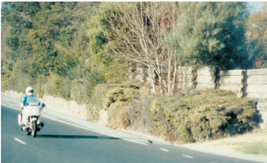
Noise barrier on top of earth mound
