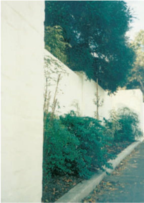
The whole wall (above) has been set back a metre or so to provide a substantial area for planting. The wall has been painted white to provide contrast with the vegetation.
