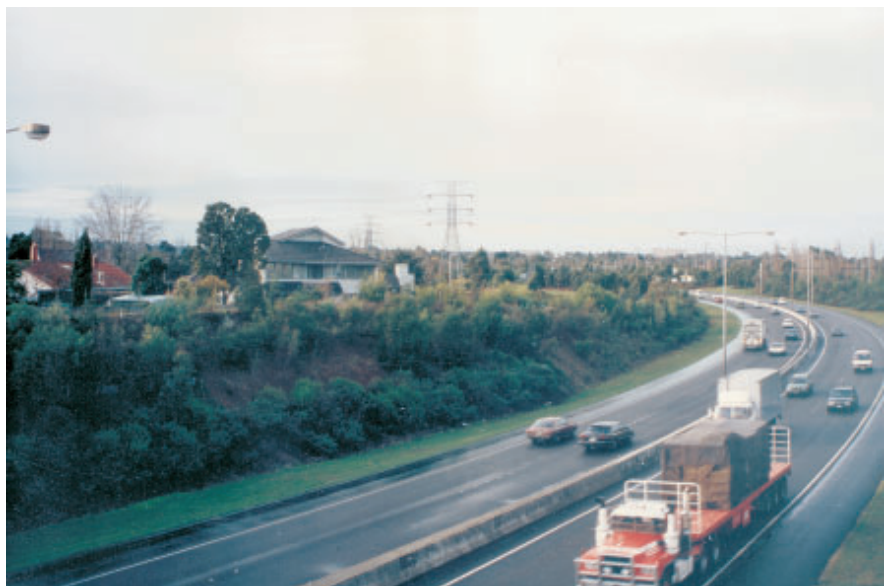
An earth mound which was built during freeway construction gives adjacent residences some shielding from traffic noise.
