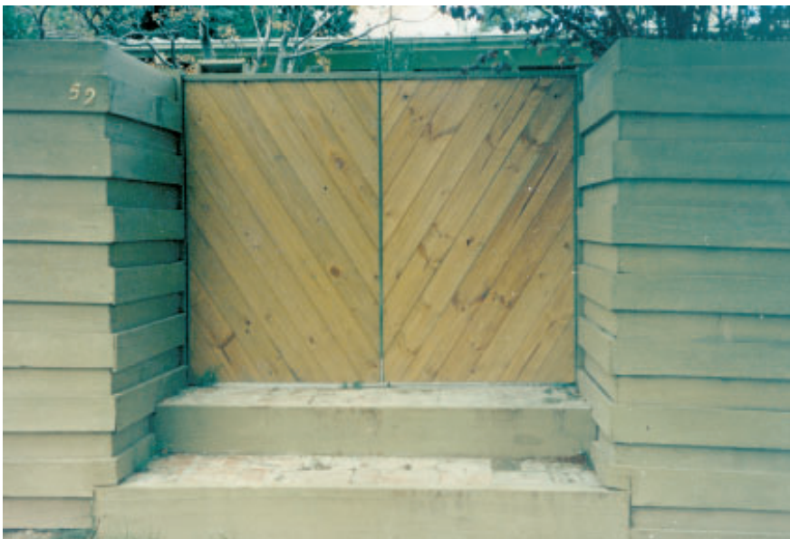
The timber fence and gate shown illustrate solid effective construction although the gap beneath the gates could be lessened.
