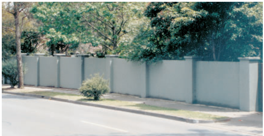
A Monolite fence consisting of wire reinforced polystyrene panels and posts, rendered with a coloured concrete and textured finish.
