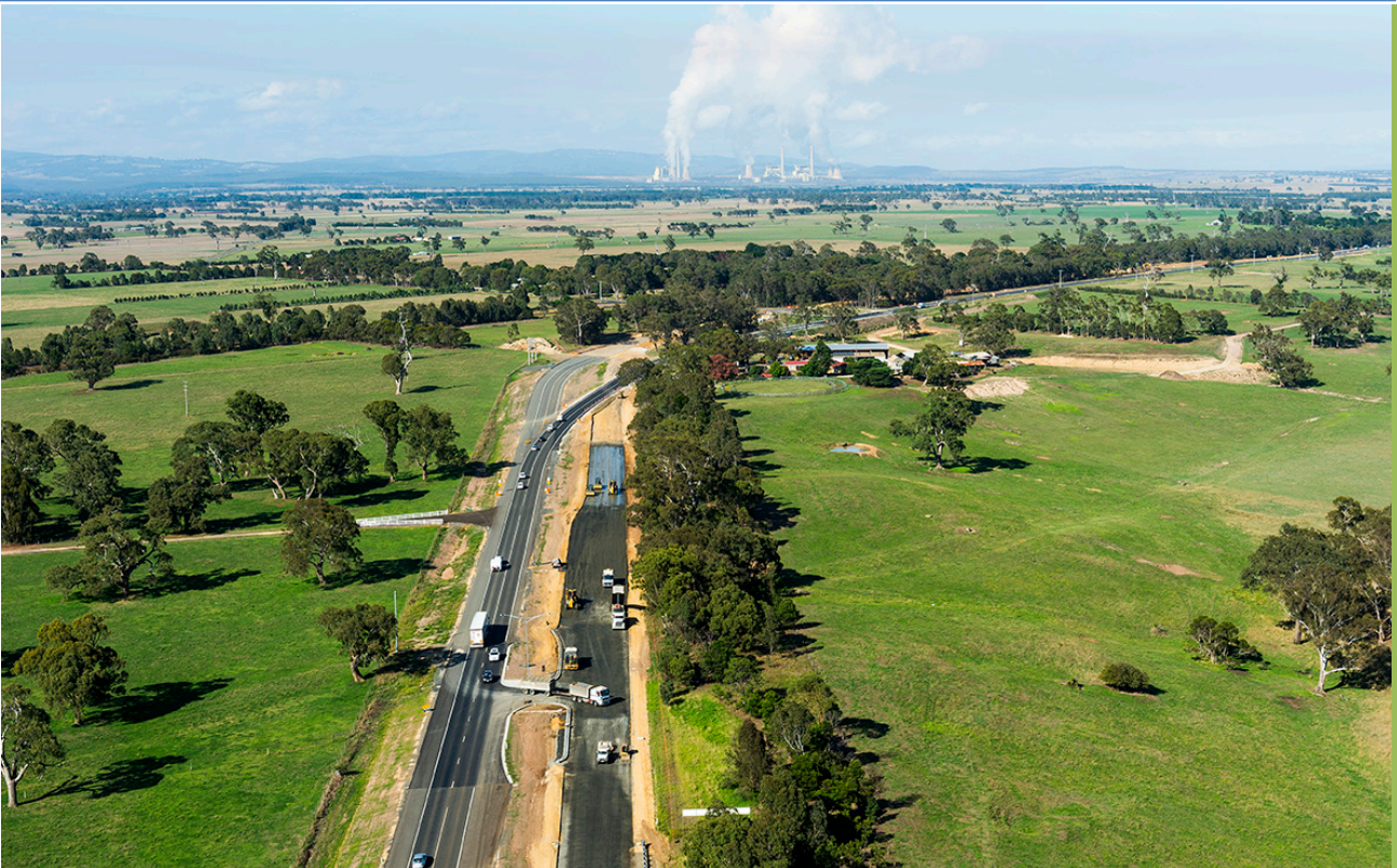
Figure 1: Aerial photograph of construction works at Flynn
