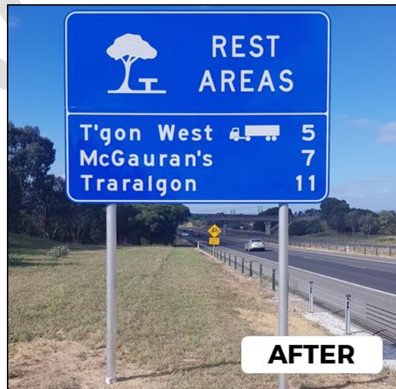
Figure – Example of a new truck rest area signage
