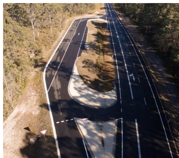
Figure 2 – Wingan River site (after)
