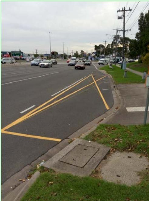
Figure 12 New line marking at bus stop to avoid confusion
