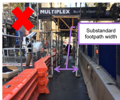
FIGURE 25: EXAMPLE OF NARROW FOOTPATH, PARTIALLY ENCLOSED
