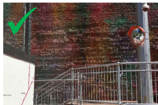
FIGURE 2: EXAMPLE OF CONVEX MIRROR USED TO FACILITATE VIEW AROUND BLIND CORNER
