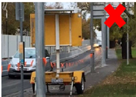
FIGURE 22: FOOTPATH BLOCKED BY VMS SIGN
