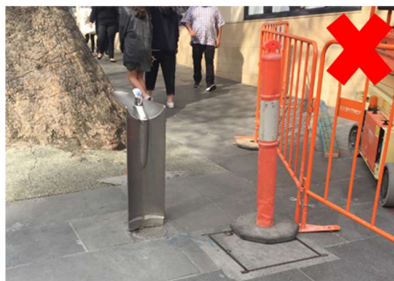
FIGURE 23: FOOTPATH NARROWED THROUGH CONSTRUCTION WORKS WITH NO CLEAR ROUTE FOR PEDESTRIANS
