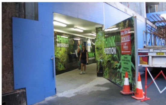
FIGURE 11 & FIGURE 12: EXAMPLE OF AGILE DIVERSION ROUTE USING MOVEABLE BARRIERS AND FENCING
