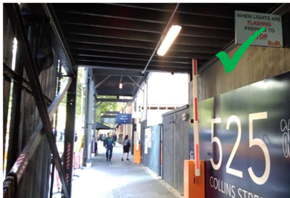
FIGURE 6: EXAMPLE OF THE USE OF PEDESTRIAN BARRIERS AROUND THE WORKSITE
