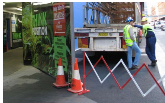
FIGURE 11 & FIGURE 12: EXAMPLE OF AGILE DIVERSION ROUTE USING MOVEABLE BARRIERS AND FENCING
