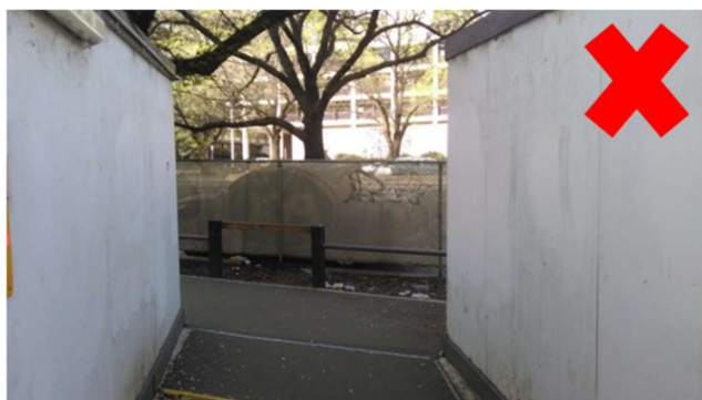
FIGURE 1: EXAMPLE OF HOARDING WITH POOR FORWARD VISIBILITY
