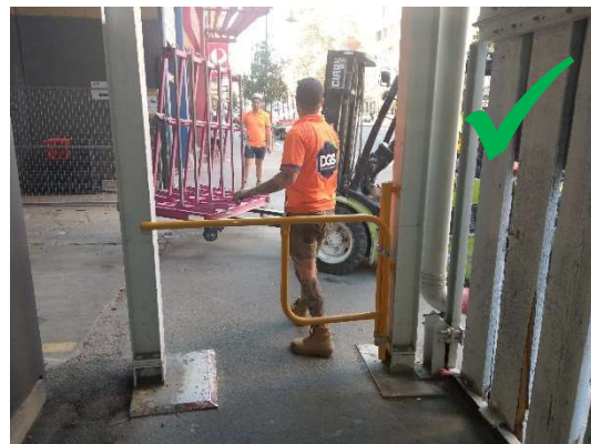
FIGURE 7: EXAMPLE OF THE USE OF PEDESTRIAN BARRIER AROUND WORKSITE
