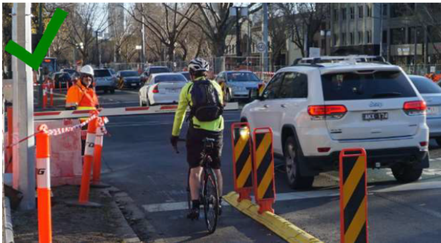
FIGURE 12: TEMPORARY BOOM GATE TRAFFIC CONTROL FOR CYCLISTS
