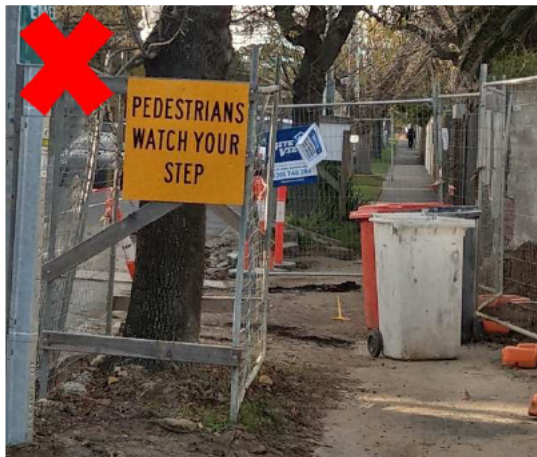
FIGURE 8: OBSTRUCTED ROUTE AND UNEVEN SURFACE - DIVERSION PATHS SHOULD BE SMOOTH AND CLEAR OF OBSTRUCTIONS
