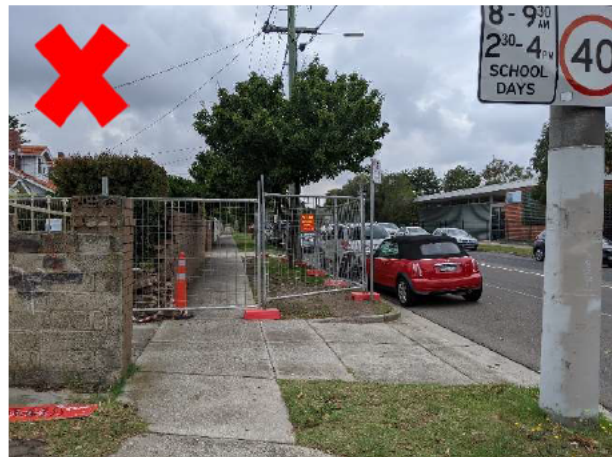
FIGURE 9: NO CLEAR ROUTE EXCEPT IN ROAD - ENSURE CLEAR, LEGIBLE ROUTES FOR PEDESTRIANS IF THE FOOTPATH IS CLOSED
