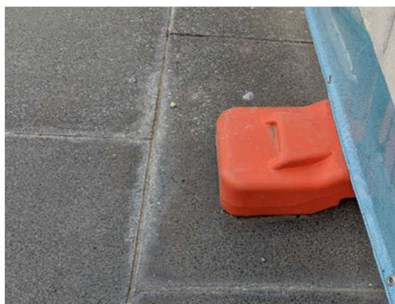
FIGURE 25: FENCE FOOTINGS CAN BE A TRIP HAZARD IN HIGH PEDESTRIAN FLOW AREAS
