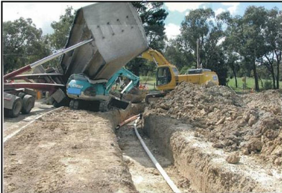
An example of what can occur if a trailer overturns. Fortunately the operator of the excavator was not in the machine at the time
