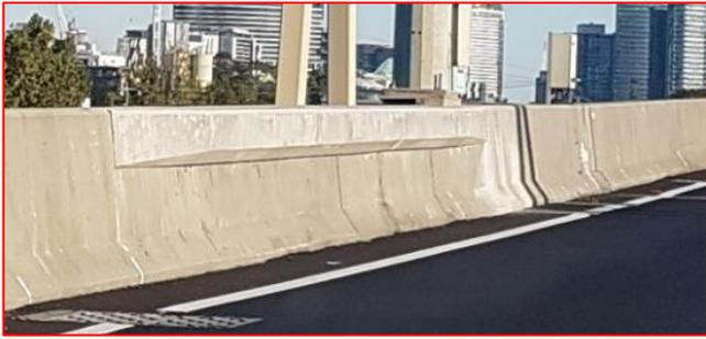
DoT does acknowledge that sway modifications can reduce vehicle roll for trucks when hazards can't be relocated or moved further back. It is critical that the balance between reducing roll and effecting passenger vehicle impacts is managed. DoT requires the modification to begin 920mm (the TL-4 height) or more above the surface level to ensure the effects to smaller vehicles are reduced. DoT recommends a 30mm maximum protrusion to minimise snag and impact severity.
