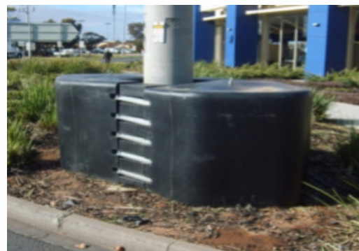
Figure 1: Typical Installation of RAPTOR Crash Cushion
