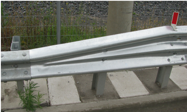
Figure 1: T-39 Thriebeam transition to Public Domain Guard Fence
