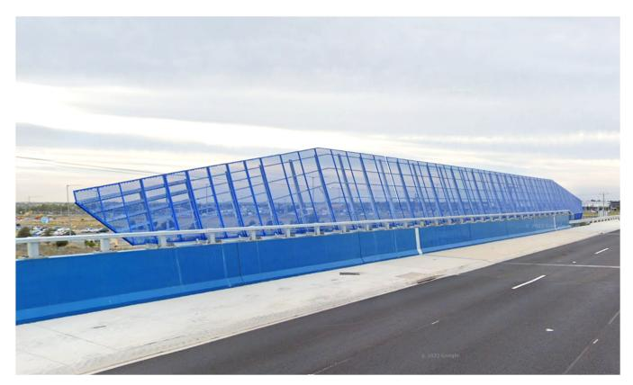
Figure 8 - Regional Rail Link, Derrimut Road - Protection Screens (Tarneit, Victoria)
