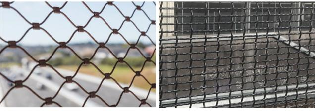
Figure 10 - Stainless steel tensile mesh (for Protection Figure 11 - Woven mesh Screen only)
