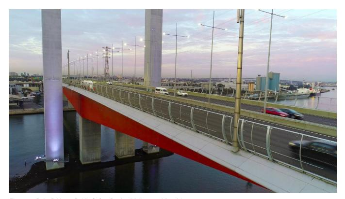
Figure 4 - Bolte Bridge - Public Safety Barrier (Melbourne, Victoria)
