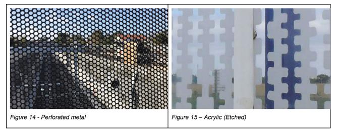
The above material examples demonstrate the different options suitable for Protection Screens and Public Safety Barriers under various conditions.
