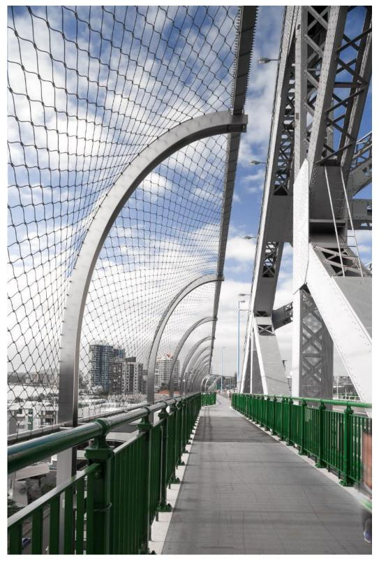
Figure 3 - Story Bridge – Protection Screens / Public Safety Barrier (Brisbane, Queensland)
