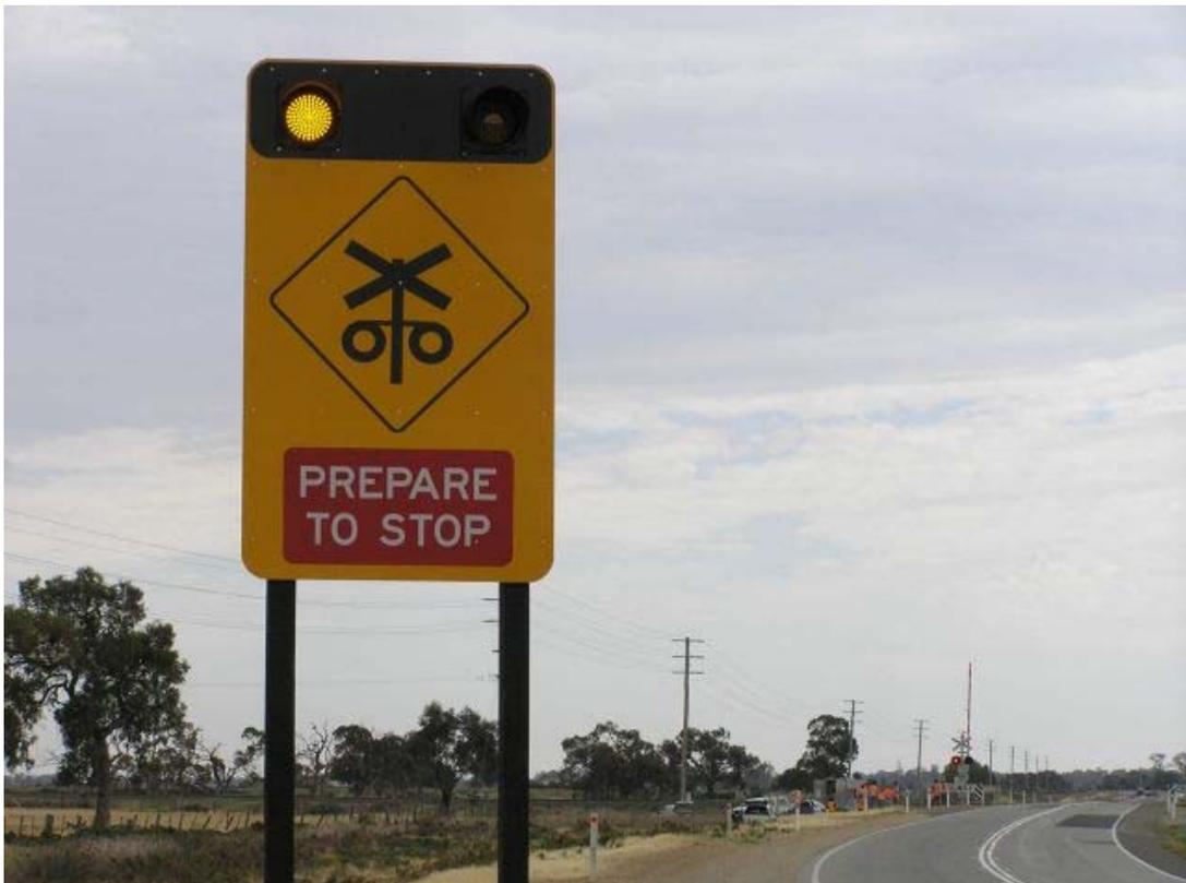
Typical AAWS sign with two yellow flashing LED lights
