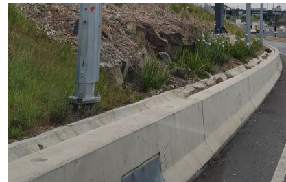
Behind concrete barrier
