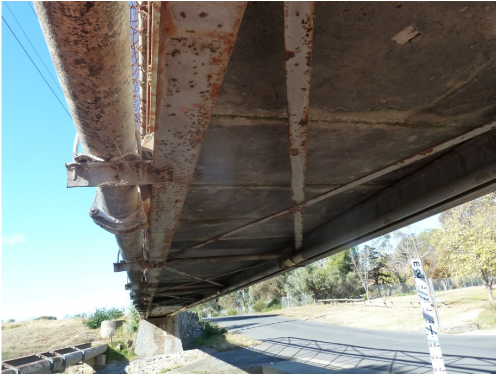
Figure 40: Surfaces damaged by spot rusting
