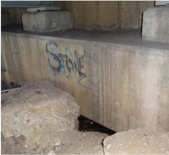
Figure 13: Cavity developing under abutment crosshead
