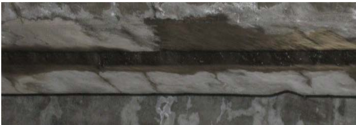
Figure 37: Shear key failure of U-Slab bridge
