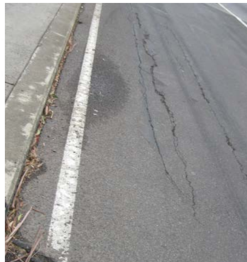
Figure 36: Shear key failure of U-slab
