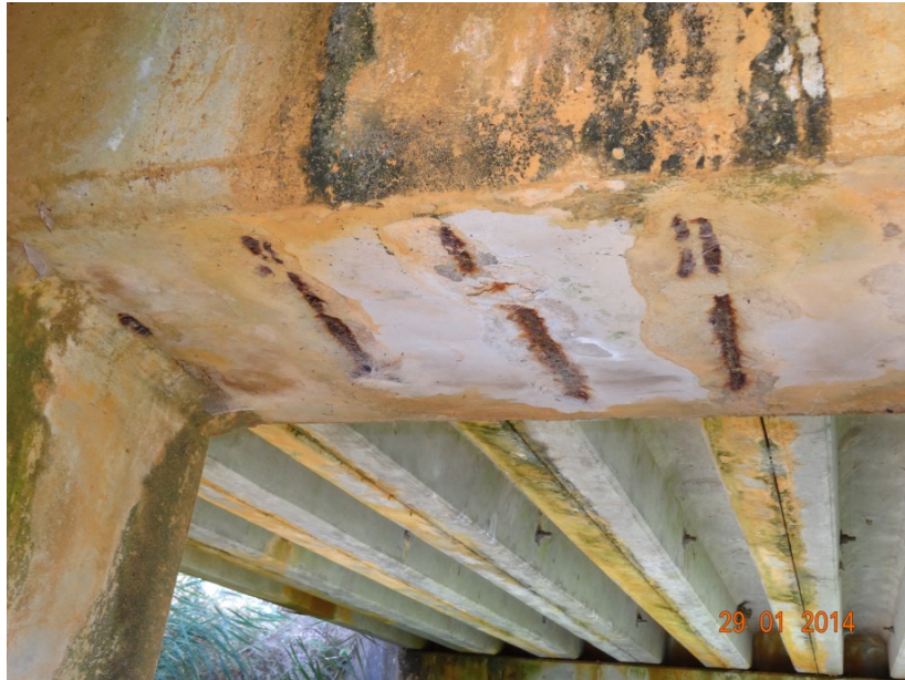
Figure 33: Reinforcement corrosion of concrete
