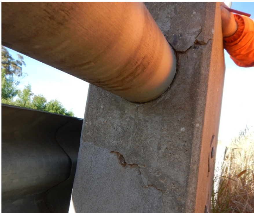
Figure 11: Steel Railing with concrete post requiring crack and patch repairs.
