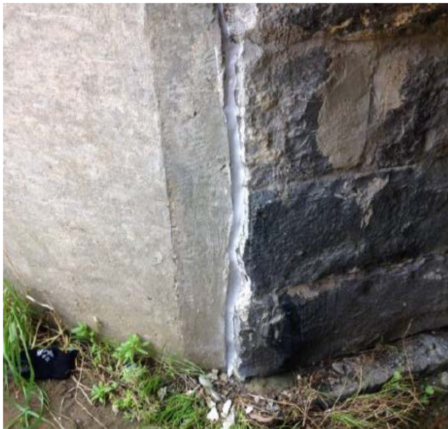
Figure 29: Active or live cracks sealed with an appropriate flexible sealant
