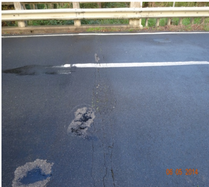
Figure 6: Potholes on the deck
