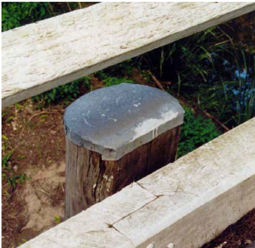
Figure 60: Flashing on pile top (RTA Timber Bridge Manual 2008)
