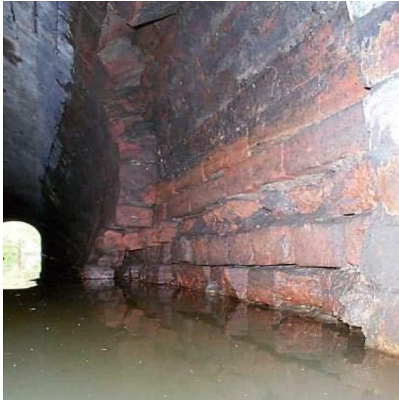
Figure 65: Missing bricks (JHR 2012)
