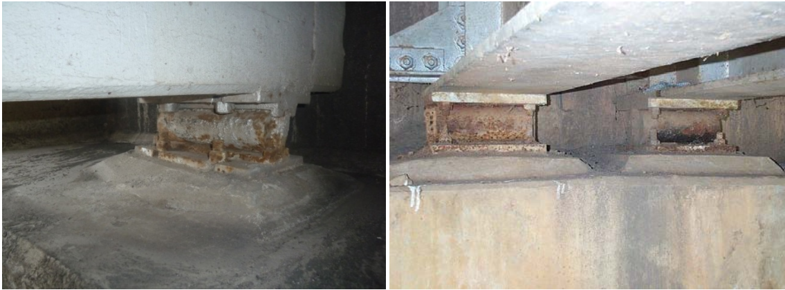
Figure 22a & 22b: Various roller bearing
