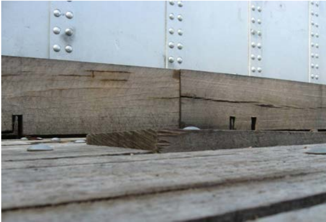
Figure 17: Loose plank needs to be retightened
