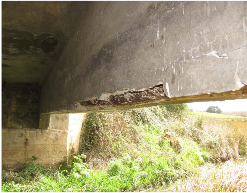
Figure 34: Severe corrosion of reinforcement
