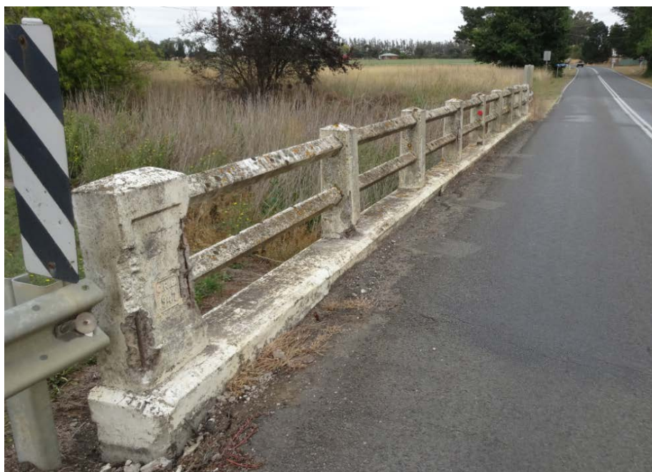
Figure 12: Concrete railing in need of repair or replacement and approach guard fence attached to parapet.
