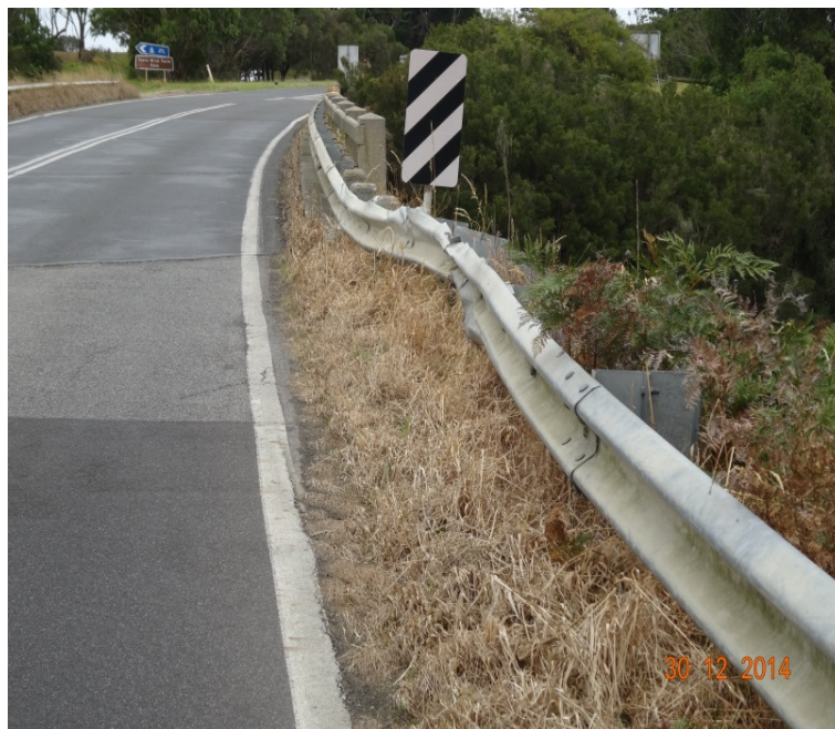
Figure 9: Damage to guardfence on bridge approach
