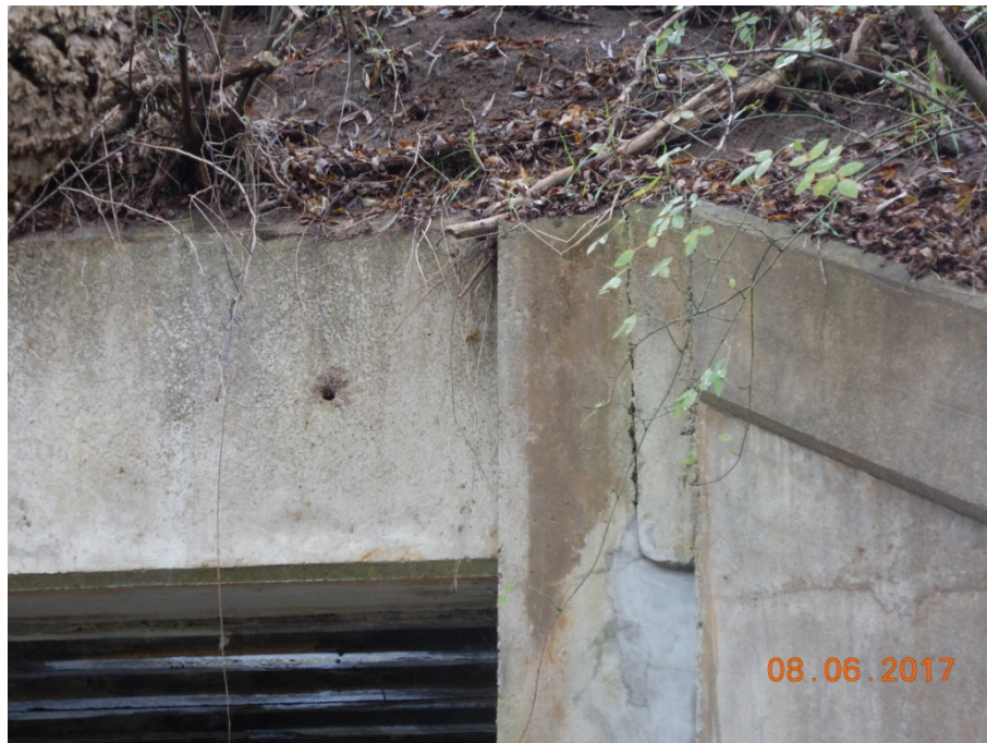
Figure 70: Wingwall cracking
