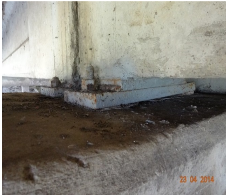
Figure 21: Sliding bearing
