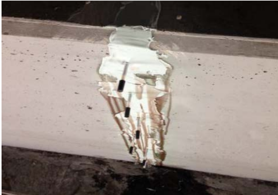
Figure 27: Injected cracks with epoxy resin through ports
