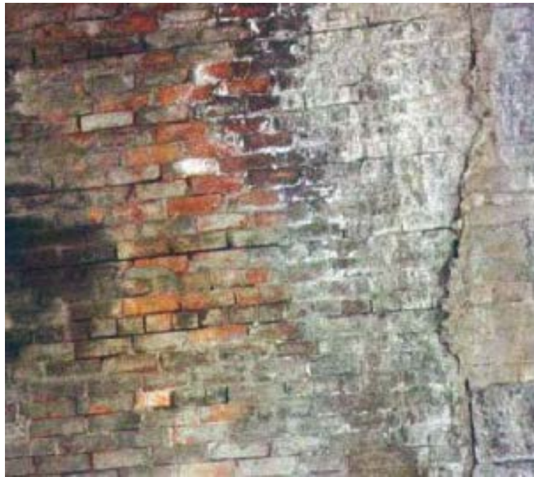
Figure 66: Cracks at sidewall and loss of mortar between bricks
