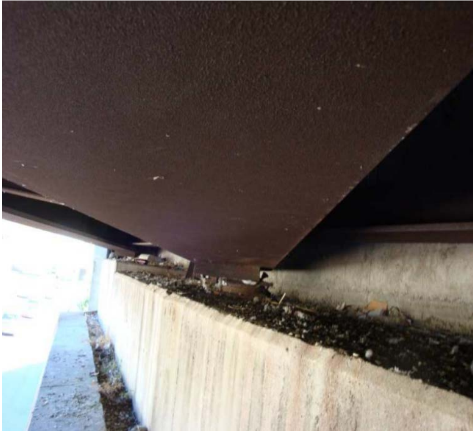
Figure 3: Abutment require cleaning
