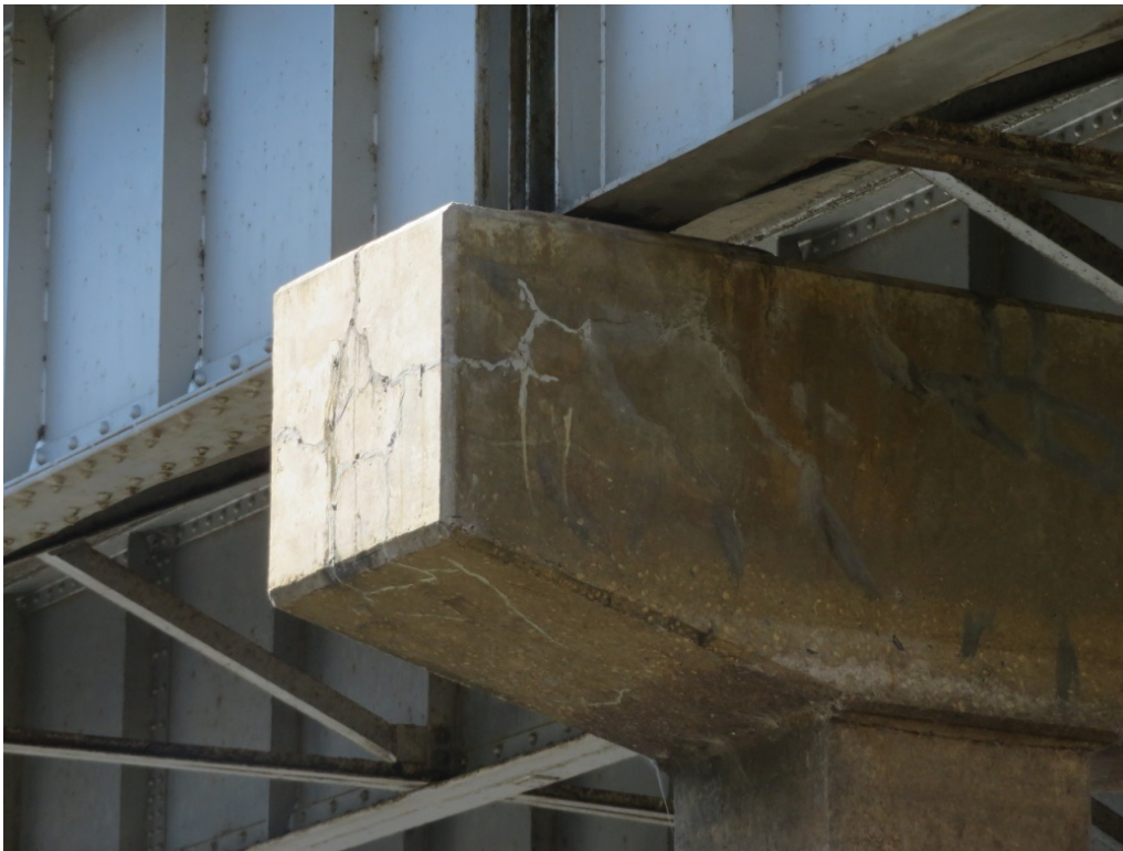
Figure 30: Cracks due to AAR
