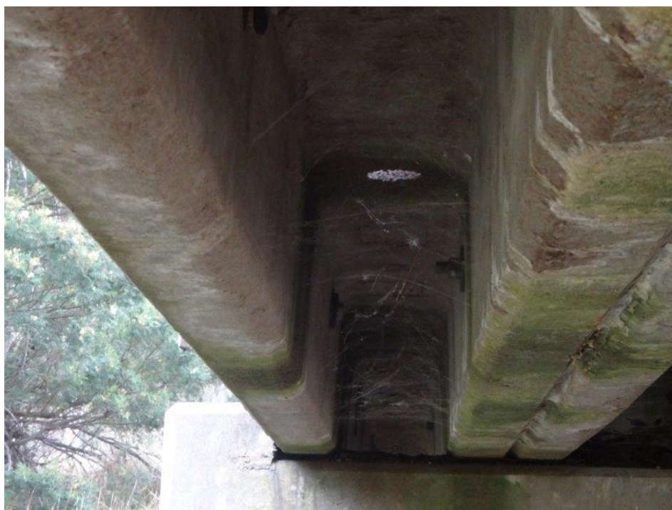
Figure 20: Scupper staining bridge beam and needs to be extended
