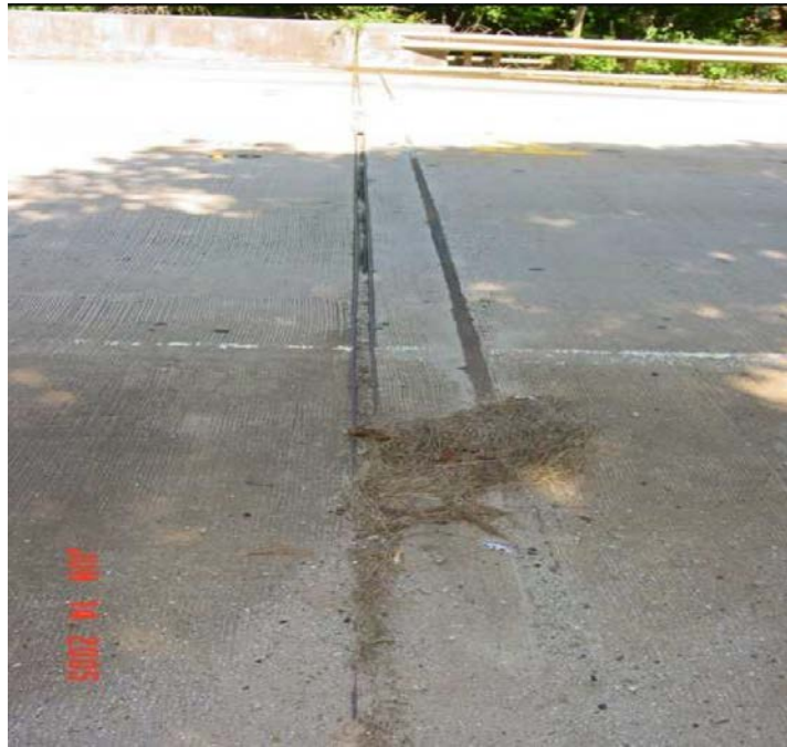
Figure 2: Deck expansion joints ( Georgia Bridge Manual 2012 )
