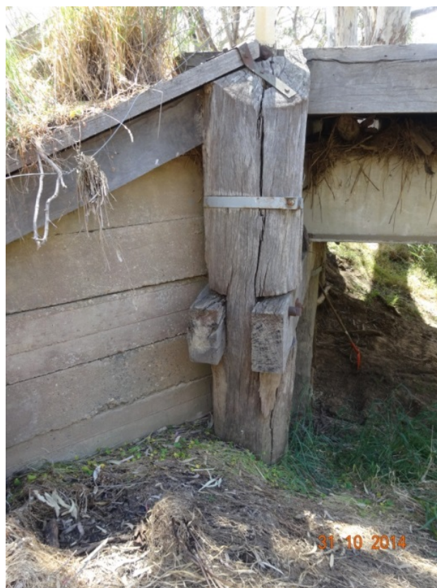
Figure 49: Splitting repair of a timber pile
