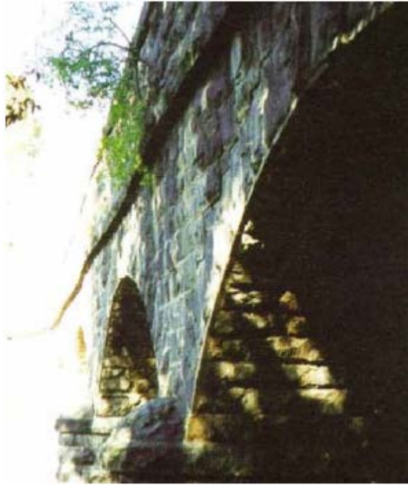
Figure 62: Vegetation growth and damaging wall
