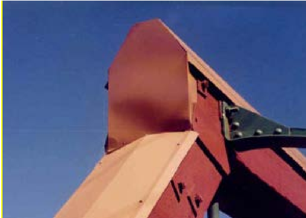
Figure 61: Flashing over timber member ( RTA Timber Bridge Manual 2008 )
