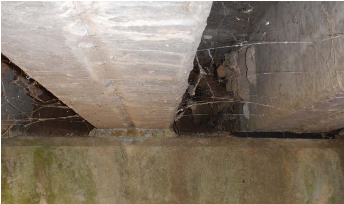
Figure 23: Mortar bearing besides a newer neoprene bearing
