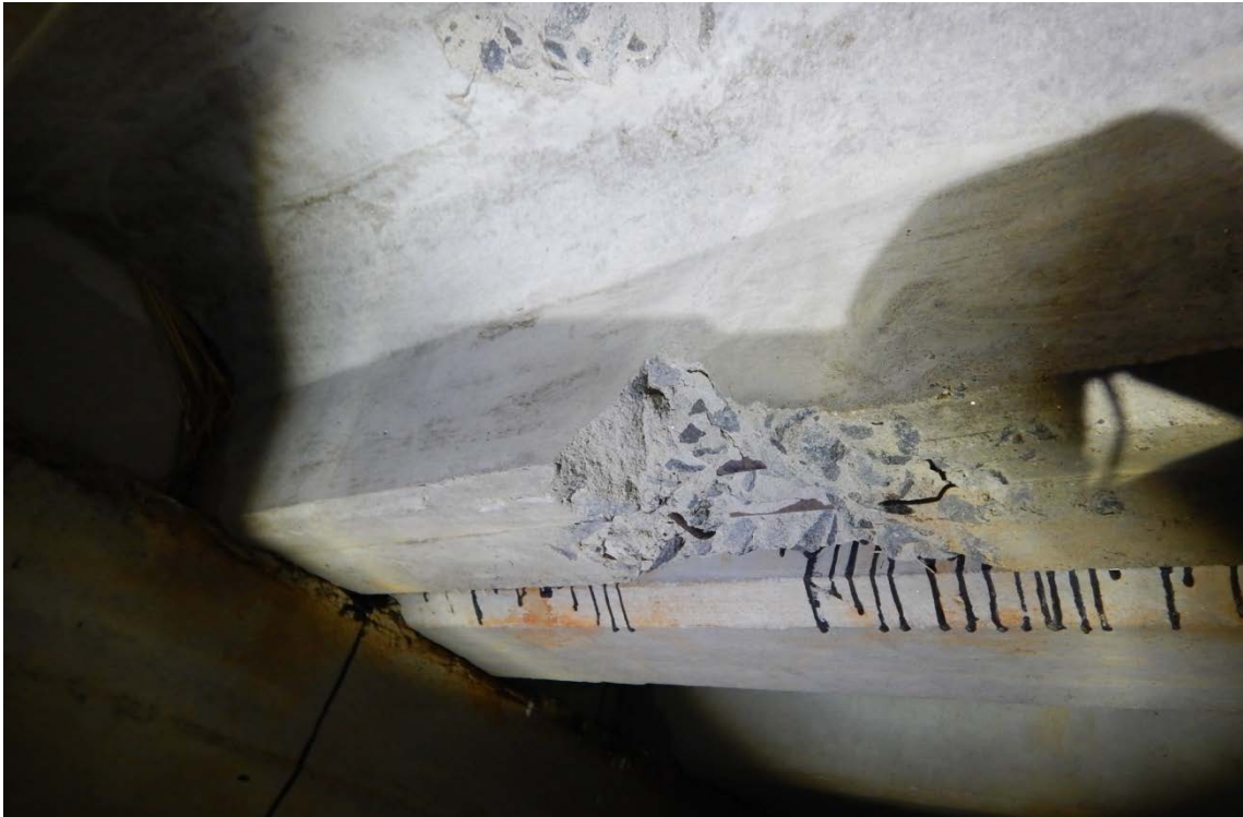
Figure 31: Spalling concrete
