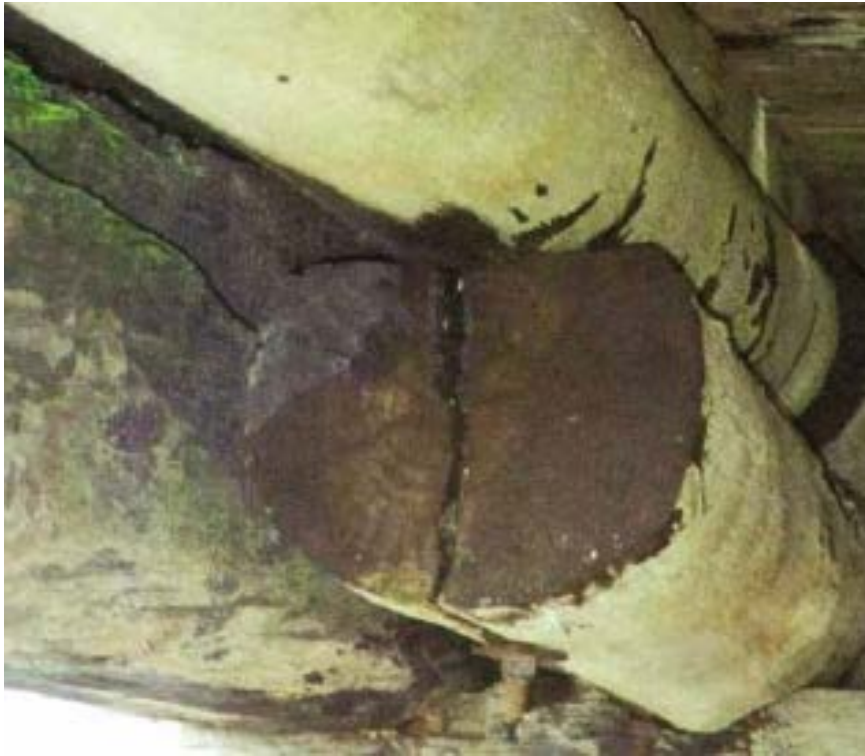
Figure 52: Split in corbel requiring anti-split bolt near the end
