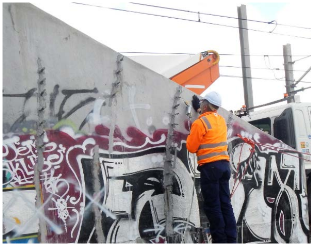
Figure 25: Crack repair - Resin injection
