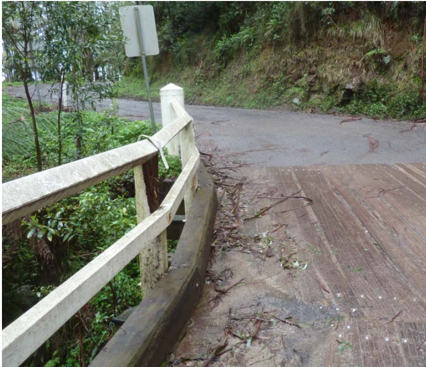
Figure 10: Timber Railing post requiring replacement.
