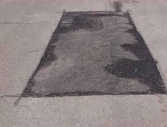
Trenches across the road that are not reinstated correctly can be dangerous for motorcyclists.
