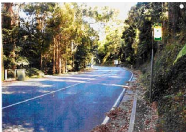
Figure 3: Where the geometry or landscape is restrictive a bus stop should not be provided.
