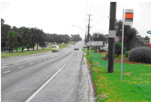
Figure 6: Narrow shoulder needs widening and sealing.
