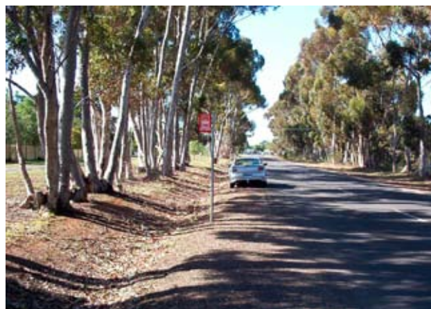
Figure 4: Where possible the bus stops should not be located near table drains
