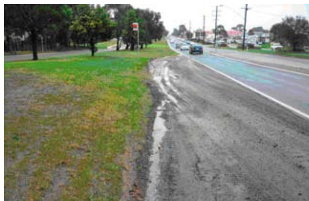
Figure 7: Bus stop does not have sufficient length after stop to allow bus to accelerate and shoulder sealing is needed.
