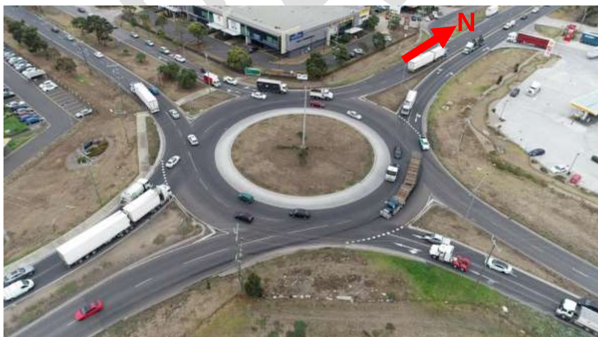
Figure B2: Drone View of Laverton survey location (view from north east)
