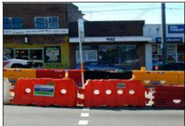
**The barrier in this photo does not provide redirective capability and can be used as a LCD only.**
