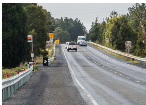
Reduced Barrier offset at a constrained location
