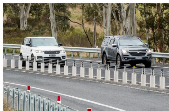
Reduced Barrier offsets for the typical cross section for median and verge barriers on a constrained site
