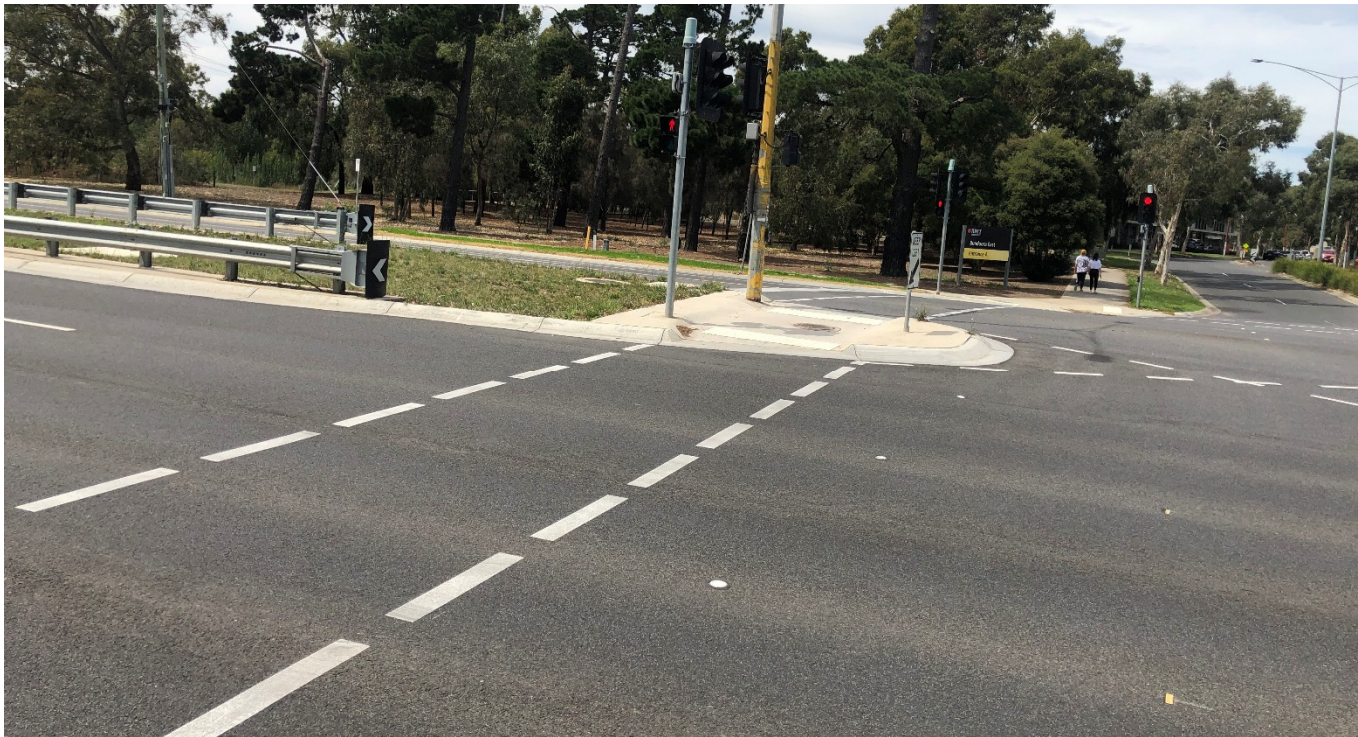
Figure 1: Example of typical signalised intersection crossing with crossing passing behind median nose
