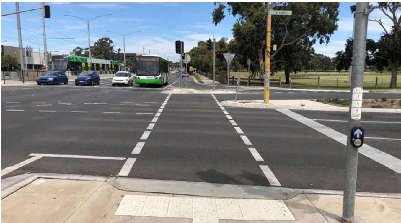
Figure 2: Example of typical signalised intersection crossing with crossing passing in front of median nose (intersections with low approach speeds and 6 lanes or less of traffic for pedestrians to cross)
