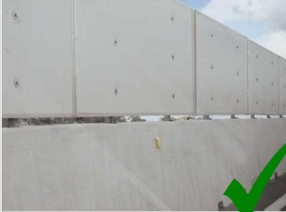
Product is neat, tidy and effective. Note that vertical alignment is achieved by correct use of stabilising wedges inside the stanchion holes. Reflectivity of panel face may require attention as per section 3.3.5 above.
