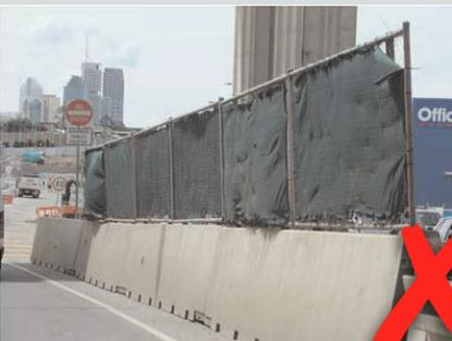
Temporary fence panels mounted on PCBs. Horizontal rails constitute a potential spearing hazard and are not permissible.
