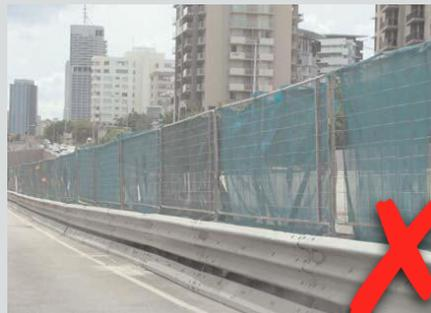
Temporary fence panels mounted on steel barrier system. It is unlikely that the method of mounting is approved by the barrier manufacturer and could compromise barrier performance. Horizontal rails constitute a potential spearing hazard and are not permissible.
