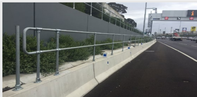
Figure C.2 – Another existing non-compliant arrangement installed to protect maintenance workers. There is no physical separation in place to suggest an errant commercial vehicle would be protected from spearing hazard.
