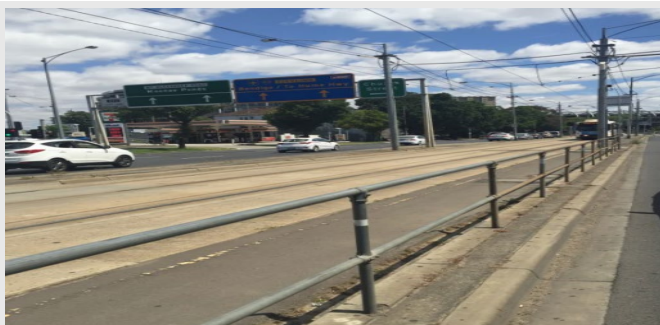
Figure C.1 – An existing non-compliant separation fence arrangement installed to guide alighting tram patrons to safe crossing points. The fencing comprises horizontal rails, which if impacted by an errant vehicle can separate or detach from the supporting posts and form a spearing hazard.
