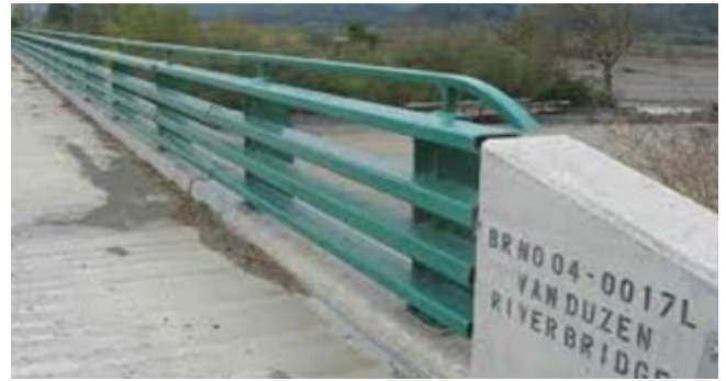
Figure 9– Pedestrian railing, a smaller longitudinal steel member welded to the rigid steel barrier.
