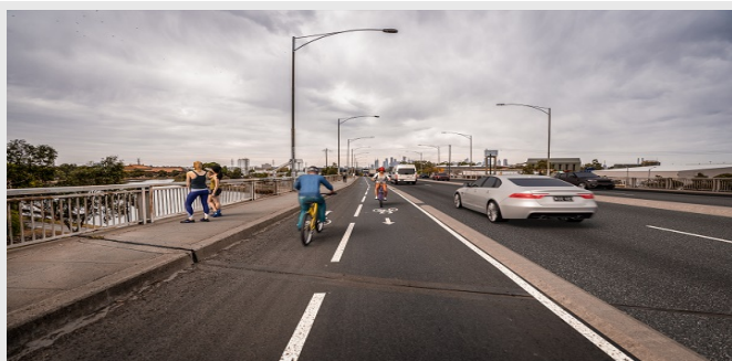
Figure A.3 – Edge treatments making use of existing kerbs and delineation to guide cyclists.
