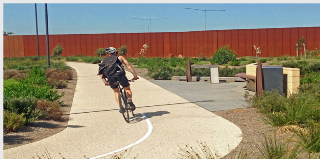
Figure A.2 – An existing path using landscaping on either side of the path and delineation on the centreline to aid cyclists around the tight curve
