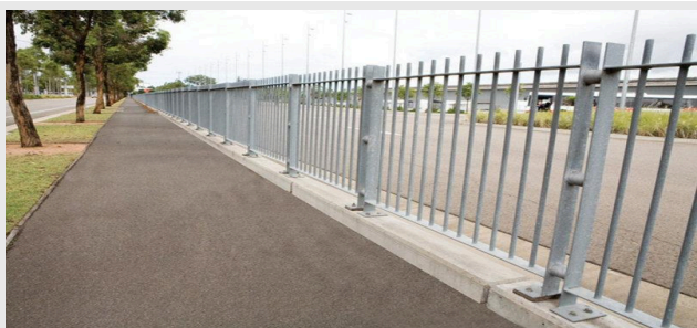
Figure C.3 – An existing non-compliant separation fence installation. The tips of the vertical bars are exposed and present an impaling risk to pedestrians.
