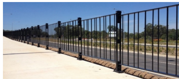
Figure 5 – Crashworthy fence, RMS (NSW) pedestrian fence
