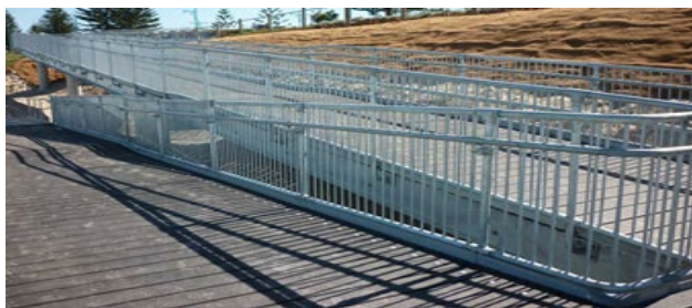
Figure 4 – Pedestrian barrier with handrail attachment
