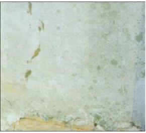
Figure 1.1.2.6 (b) Spalling of concrete
