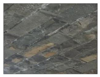
Figure 1.1.5.4 Dropping arch masonry block
