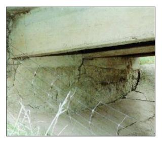
Figure 1.1.2.2. Disintegration of concrete
