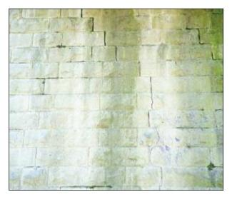
Figure 1.1.5.1 Cracking through masonry
