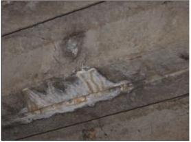
Figure 1.1.2.9 Efflorescence on the beam soffit
