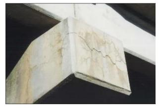
Figure 1.1.2.8 Alkali aggregate reaction (AAR)
