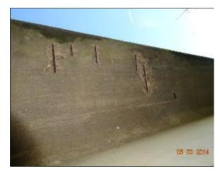
Figure 1.1.2.6 (a) Spalling of concrete
