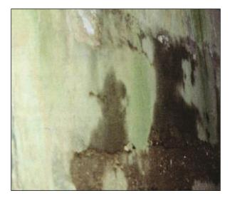
Figure 1.1.2.1. Scaling of Concrete
