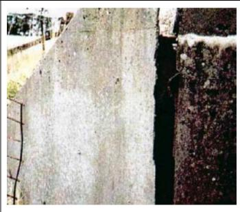
Cast-in-situ wingwall moved well away from abutment wall with loss of embankment fill from behind.
