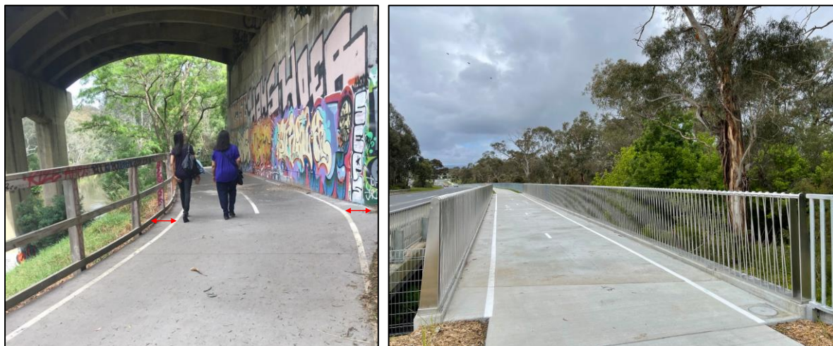
Figure V5.8: Examples of Off-Road Path Edge Linemarking to Hazards
