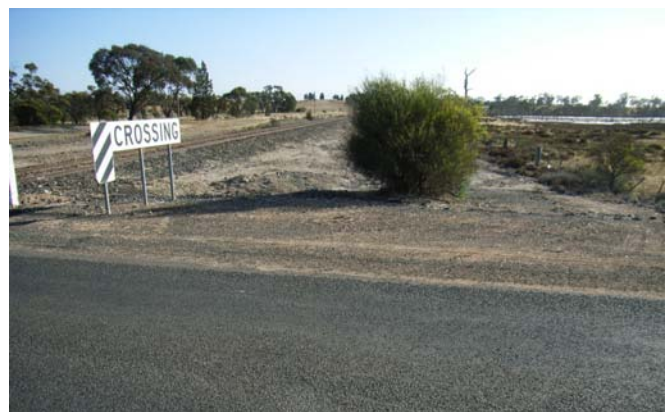
Figure VA2.3: Obstruction in the Sight Triangle at the Stop Line
