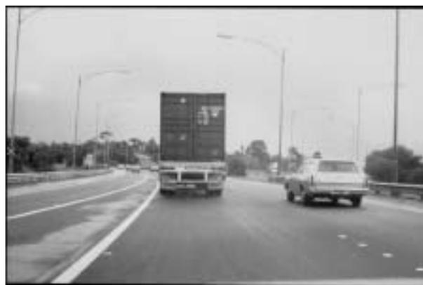
*Reduction in water spray after placement of OGA*
