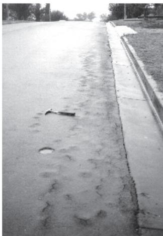
Acid salt induced damage to untrafficked pavement edge
