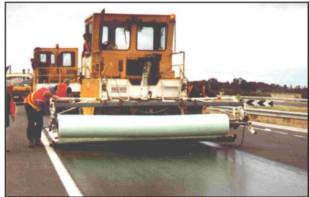
Figure 1 Fabric spreader attached to multi wheel roller
