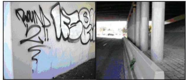
Fig. 1 Repeated painting out of graffiti, previous markings bleeding through (L), Long life anti-graffiti coating typically 3 m above ground level (R)
