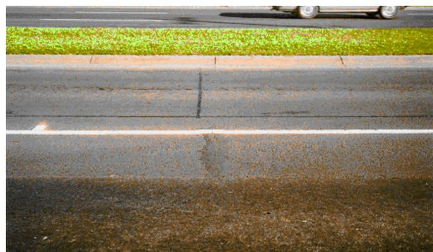
Transverse cracking in "saw cut and seal" joints. Note the reflective cracking does not extend into the BSRA section (foreground).
