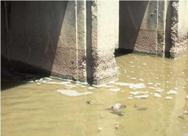
**Figure 1: Concrete bridge pier damaged by acidic runoff from ASS.**
