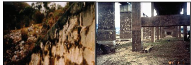
Fig. 2. Cracking due to alkali aggregate reactivity and related dampness (L), Crack Injection and Application of Flexible Epoxy Coating for ASR Repairs (R)
