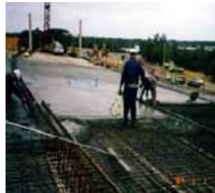
Fig 3 - Application of evaporative retarder
