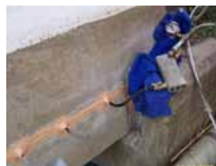
Fig 7 - Injected cracks with epoxy resin through nipples
