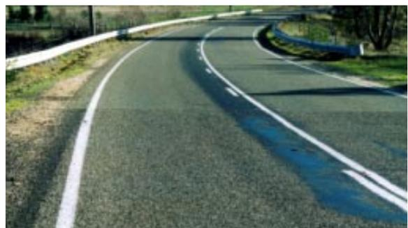
**Figure 1 Flushing along the centre-line as a result of patching too close to resealing**
