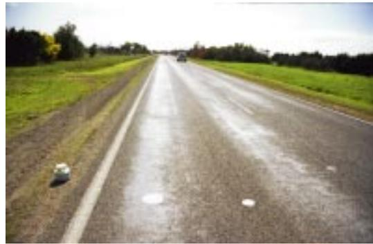
Figure 2 Wheelpath flushing
