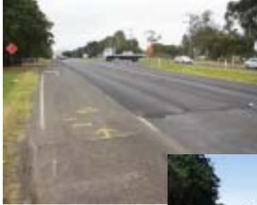
Regulation prior to placement of geotextile reinforced seal.
