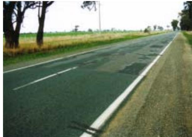
Bituminous surfacing treatment on a rural road using a regulation followed by a geotextile reinforced seal
