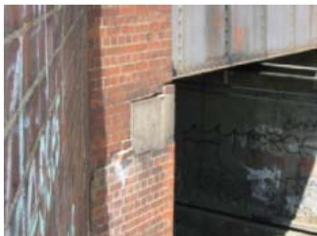
Fig. 2 - Traffic vibrations in the steel beam could have caused the crack
