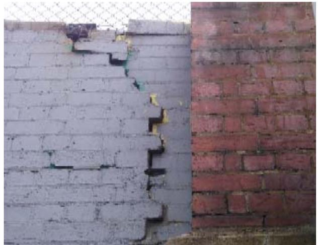
Fig. 7 - Severe cracking of wall due to settlement and pressure from behind
