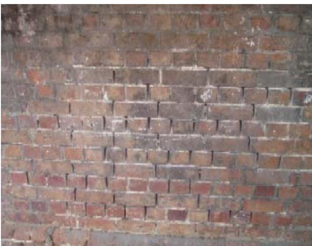
Fig. 11 – Extreme loss of weak jointing mortar, which requires refilling and repointing
