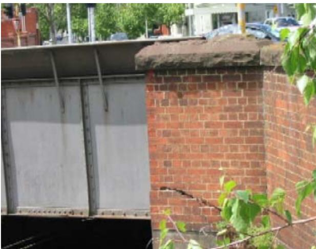
Fig. 5 - Cracking in the brick pylon from the interaction of blue stone capping and steel beam
