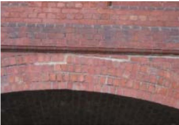
Fig. 3 - Horizontal crack on the crown of the arch.
