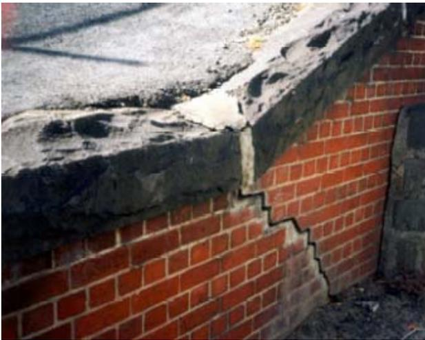
Fig. 10 – Diagonal cracking caused by movement
