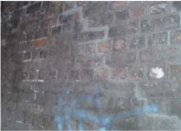
Fig. 9 – Repointing of diagonal cracking on dirty wall
