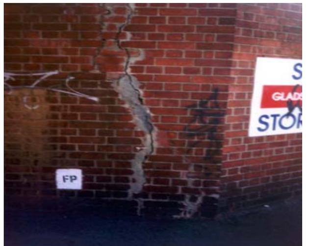
Fig. 8 - Diagonal cracking due to movement and pressure from behind. Failed repointing work
