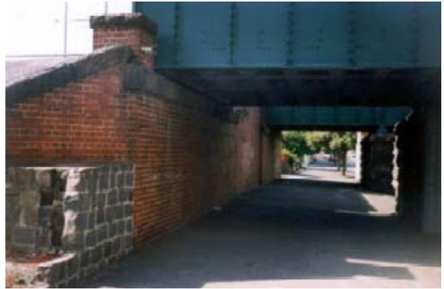
Fig. 12 – Typical combination of brick walls, bluestone capping and steel beams
