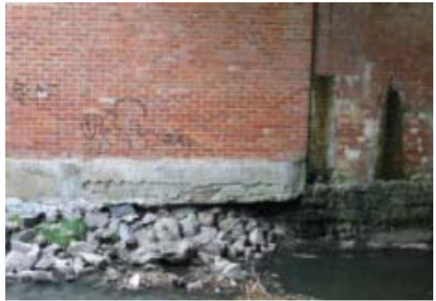
Fig. 6 - Scour at the base of abutment wall needs restoration
