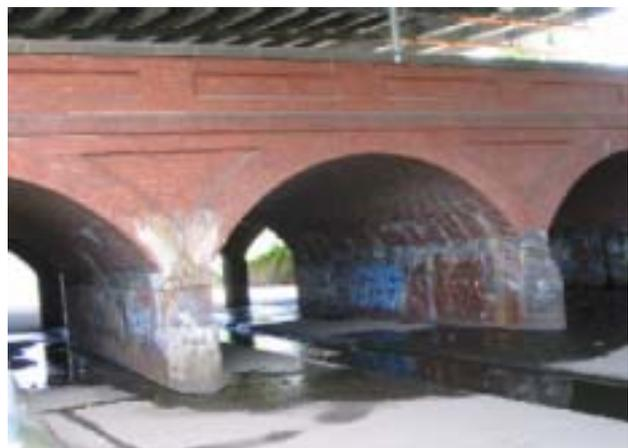
Fig. 1 - Efflorescence and leaching on brick work due to water moving down from above
