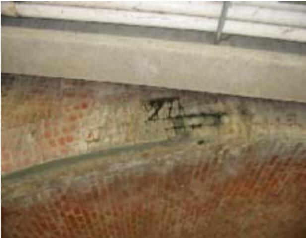
Fig. 4 - Water seepage through the arch. Source of percolating water from the road above
