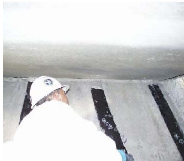
Fig. 2 Placement of the FRP with correct orientation and placement tolerances
