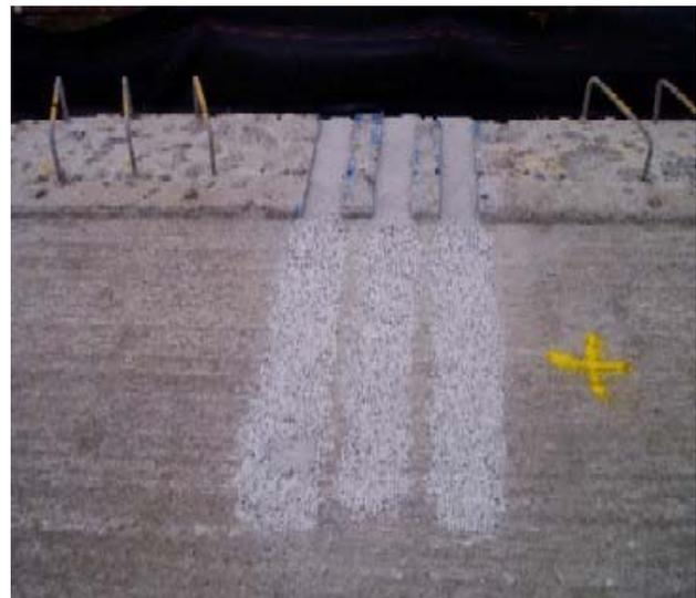
Fig. 1 Preparation of the concrete substrate with acceptable surface roughness
