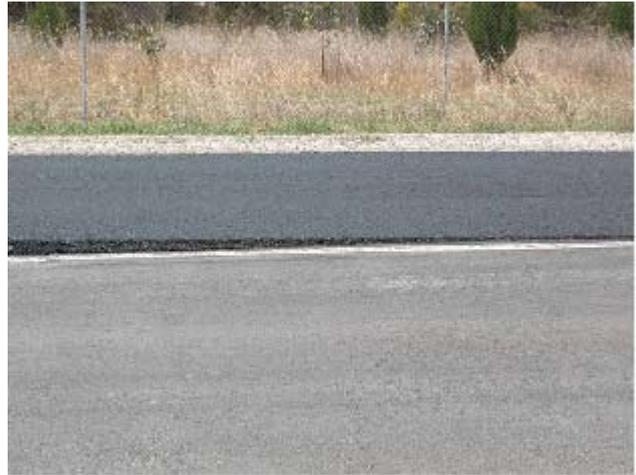
*Final result after use of averaging beam to correct longitudinal shape*
