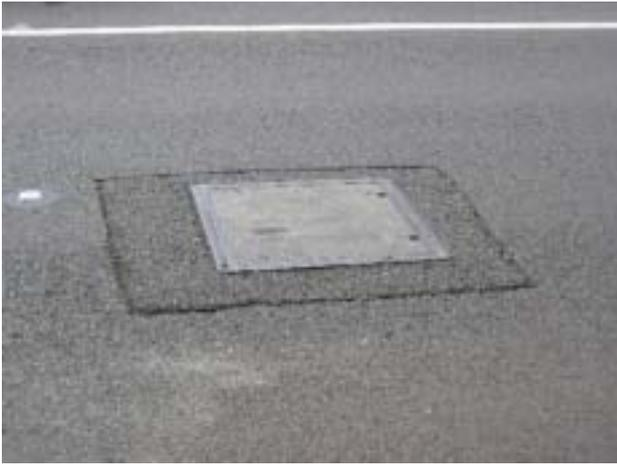
*Filling around manhole after asphalt has been placed rather than before placement*
