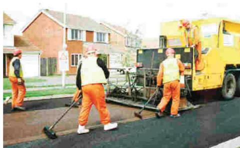
Figure 2: Placing slurry surfacing
