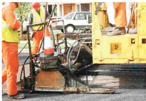
Figure 1: Slurry surfacing spreader box
