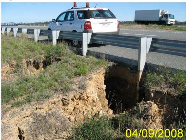
Figure A5: Cavity created by piping.
