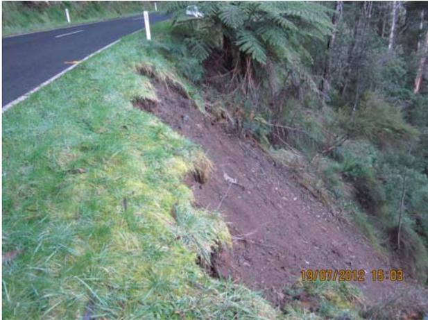
Figure A3: Slumping of soil.
