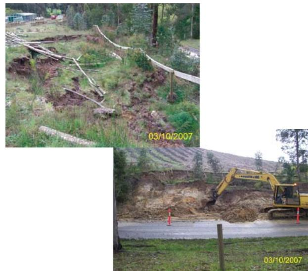
**Figure A2: Rotational failure.**
