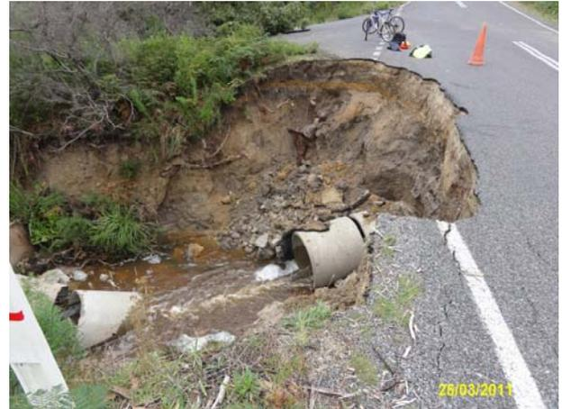
Figure A6: Erosion at culvert outlet
