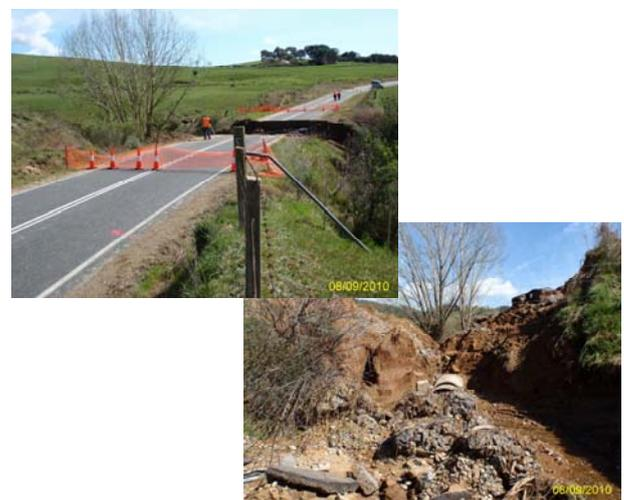
Figure A7: Embankment fill acting as a dam.
