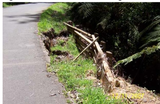
Figure A8: Failure of minor retaining wall.
