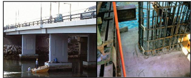
Fig. 1 Bridge in marine environment (L). Location of Macrocell/galvanic current corrosion monitoring probes within column at various levels (R)
