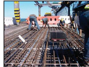
Fig. 2<sup>(8)</sup> Installation of an anode into new concrete member as part of cathodic prevention
