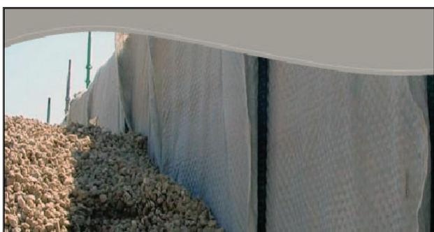
**Figure 4. Drainage provision over the entire face of a structure**
