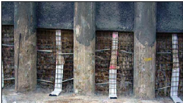
**Figure 3. Drainage line behind retaining panels**
