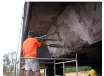
Fig 4 - Removal of cores from fire damaged concrete
