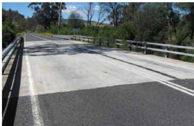
Figure 1: Concrete wearing surface
