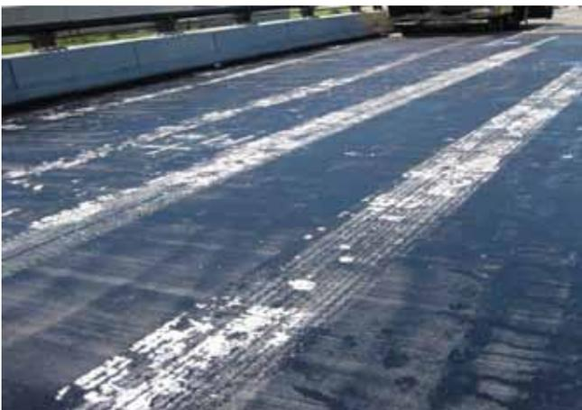
Figure 2: Pick up of prime by construction traffic
