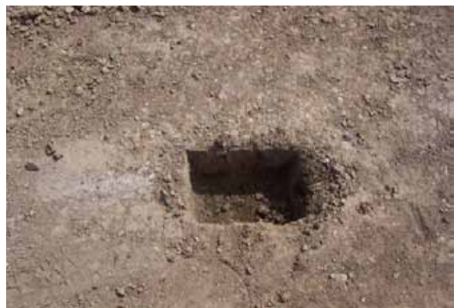
Figure 11 Appropriate sampling from the road for moisture content and other laboratory tests
