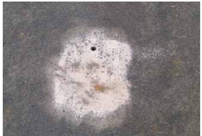
Figure 8 Test site, showing access hole, with sand spread to minimum thickness, after sweeping to remove loose material
