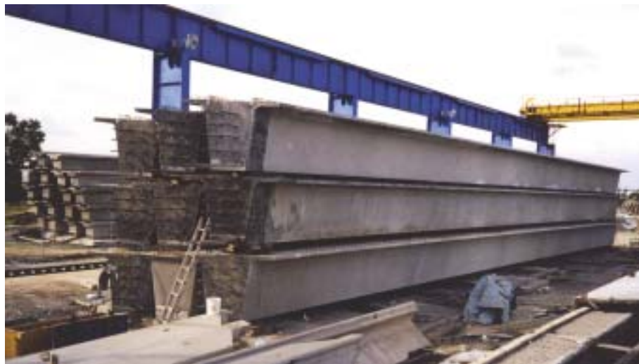
Figures 5.1 Surveillance checklists will include observation of lifting and storage methods, such as the storage of completed beams, pictured here in the casting yard.
