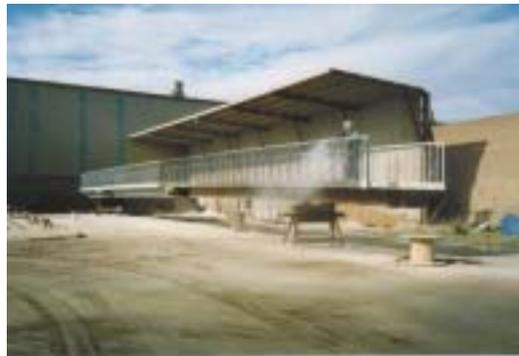
**Figure 2.1:** *Dry abrasive blasting is often an open-air activity. The Surveillance Officer should obtain verification that ambient conditions were suitable and recorded, and that prepared surfaces were not adversely affected by moisture or salt contamination prior to coating.*
