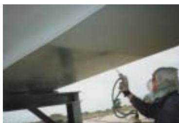
***Figure 6.1: The Surveillance Officer should verify that the required surface preparation has been achieved, the coating is applied within the allowed time, and that coating application has been to the manufacturer's instructions***
