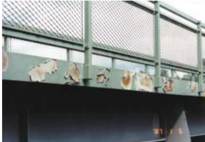
**Figure 7.1:** *Surface preparation which is below the minimum required, or the omission of primer or intermediate coating, or coatings which are below the thickness specified, may lead to premature failure of the coating system.*
