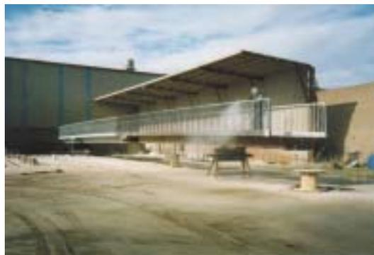
**Figure 6.3:** *Dry abrasive blasting is often an open-air activity. The Surveillance Officer should obtain verification that ambient conditions were suitable and recorded, and that prepared surfaces were not adversely affected by moisture or salt contamination prior to coating.*
