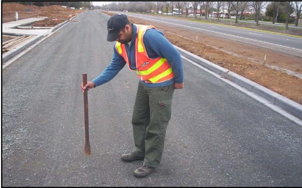
**Figure 9 : Mattock Pick used to Test Hardness**
