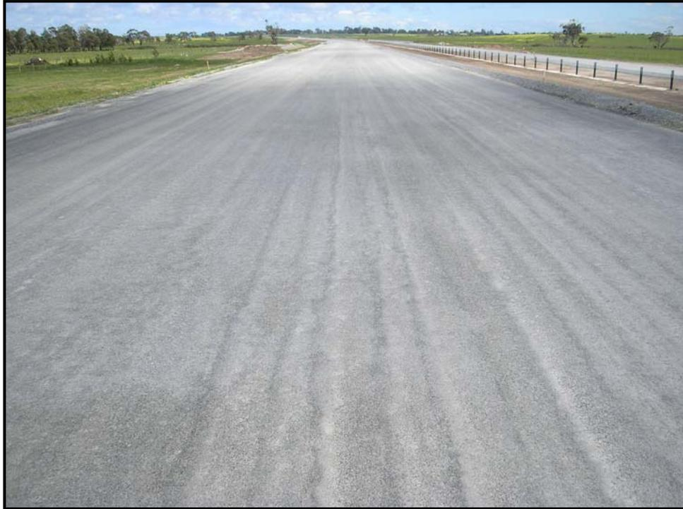
**Figure 8 : Excessive Slurring of Fines**
