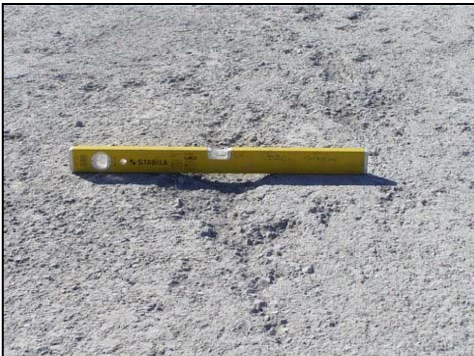
**Figure 5 : Tearing of Pavement - Ravelling**
