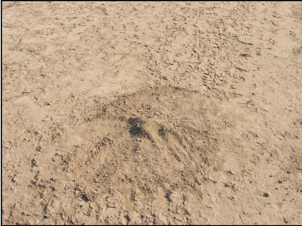
**Figure 2 : Layer of Fine Material on Top of Crushed Rock**
