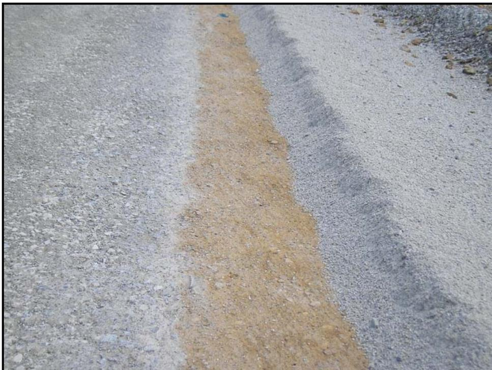
**Figure 3 : Excess Material Swept from Compacted Layer**
