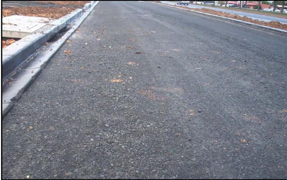
**Figure 7 : Loose and Foreign Material at Surface**
