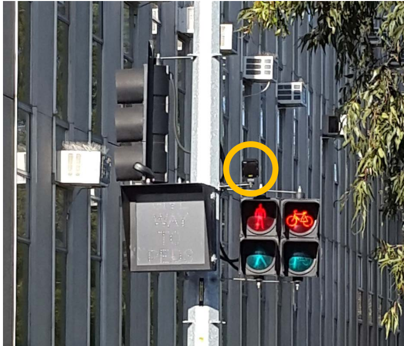
Figure 16: Puffin detector located above pedestrian signal (circled).
